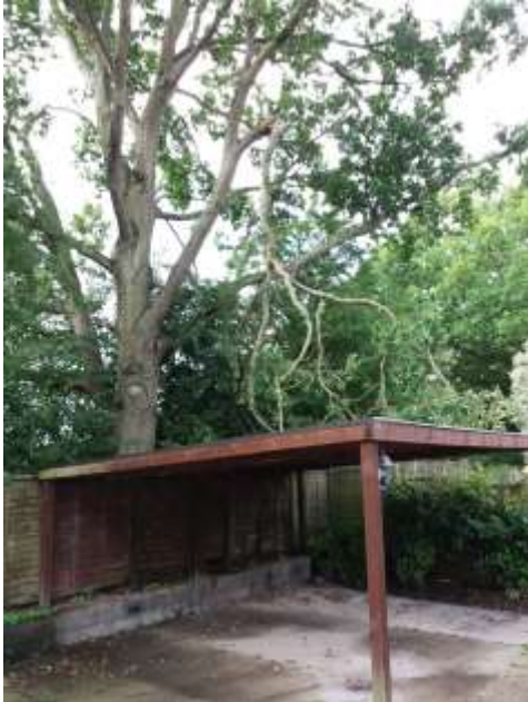
Failed oak limb hanging over a car port in North Baddesley (Amelia Williams)
