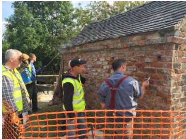
Volunteers learning traditional brickwork techniques on a Caldon Canal lengthsman's hovel
